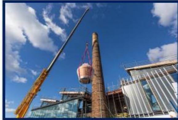
Construction of the new Rosebank Distillery
